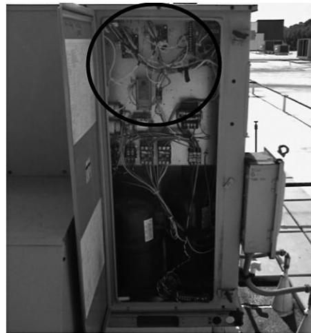
Model PACE2 retrofits with optional return-air sensor kit, installed in package unit control panel. Photo courtesy of PaceControls LLC.
